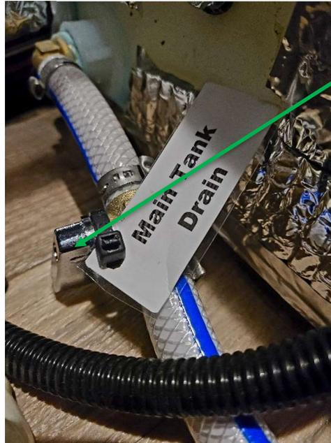
Leave valved closed (as shown in picture) unless you are manually draining your main water tank
