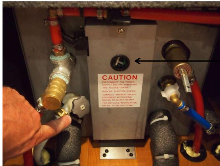
The reset button is located on the water heater unit, accessible through the small hole on the front panel of the water heater shown in the above picture.
