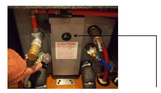
The <u>reset button</u> is located on the water heater unit, accessible through the small hole on the front panel of the water heater shown in the above picture.
