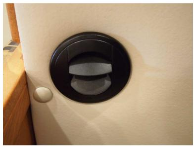
You should clean the unit's air filter at least twice a month. To remove the air filter simply remove these four screws, rinse the filter clean, and/or replace it. Note that if your sleeper has an auxiliary unit, it uses a sock filter in place of an enclosed filter.
