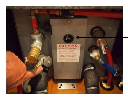
Try to remember not to engage the lighted water heater switch while the engine block is still hot; by doing this, you take the risk of tripping the reset breaker on the thermostat of the water heater. The <u>reset button</u> is located on the water heater unit, accessible through the small hole on the front panel of the water heater shown in the above picture.
