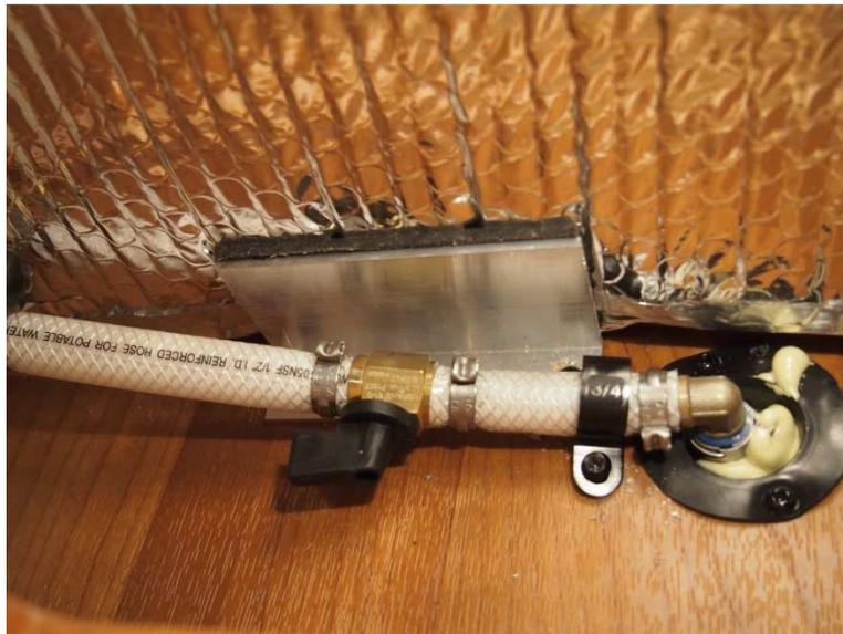
3. Make sure the valves close to the water screen are open. It is unlikely these valves will be closed.
